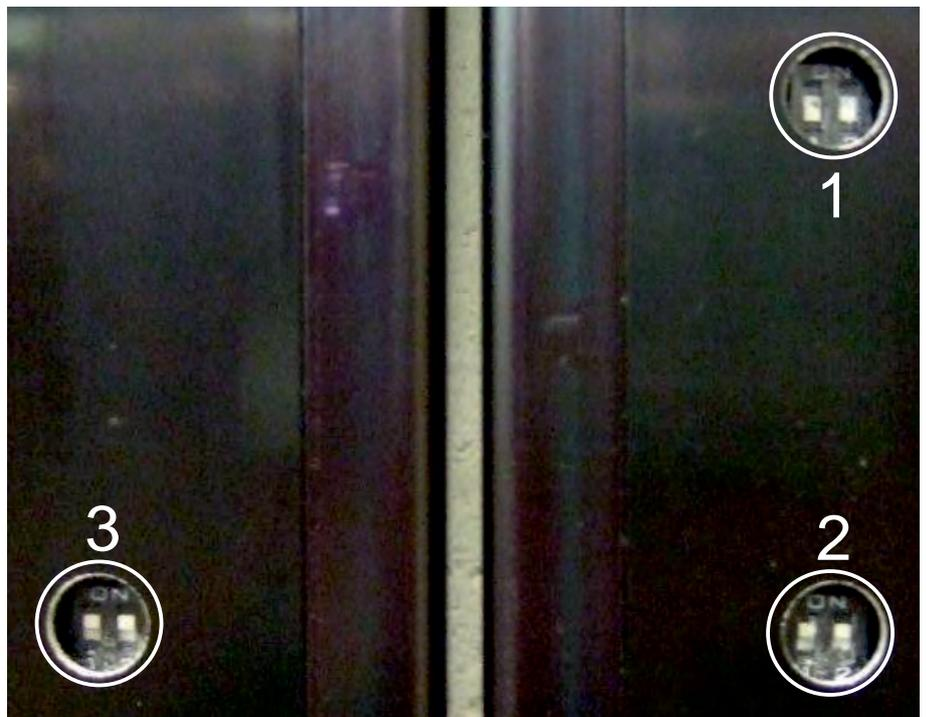
2 & 3: Both Rx and Tx have SILL light and BPL master controls. Switch 1 controls SILL and switch 2 controls the BPL light. Each can be turned on or off as required. The default delivery settings have both set to the on positions
